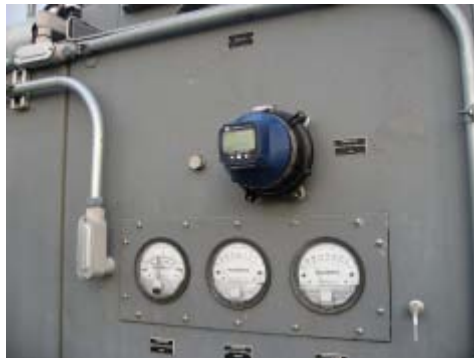
Wireless Magnetic Reader Monitors Filters and Airflow
